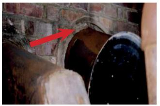
The content of asbestos is 100% unless combined with other fibres. The material is liable to degrade if exposed to the atmosphere and also likely to become more friable with age. *Asbestos flashguards*
